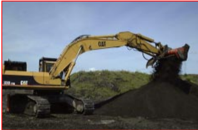
An ALLU SM4-17 (attached to a Cat 330) working with top soil.
